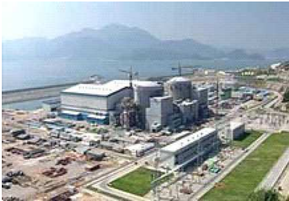
Figure 44: The overview of the Lingao nuclear power reactors
