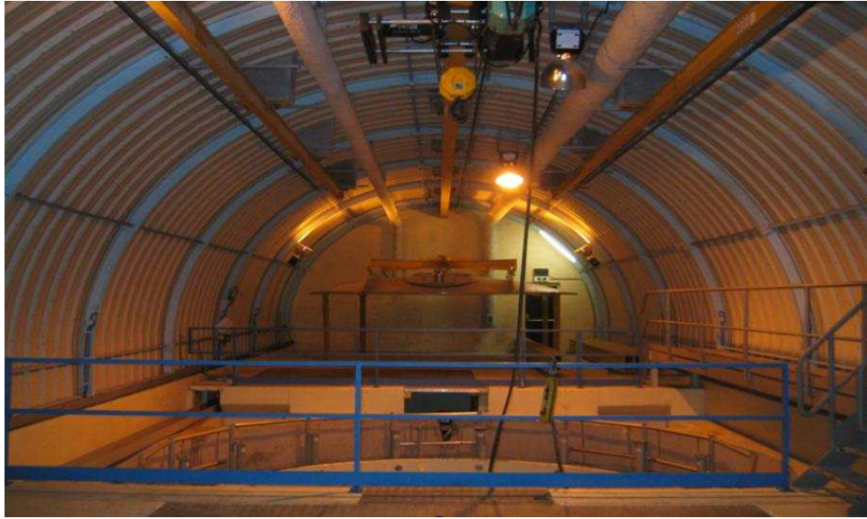
Figure 3.3: Picture of the CHOOZ-far detector site taken in September 2003. The original CHOOZ laboratory hall constructed by EDF, located close the the old CHOOZ-A underground power plant, is still in perfect condition and could be re-used without additional civil engineering construction.
