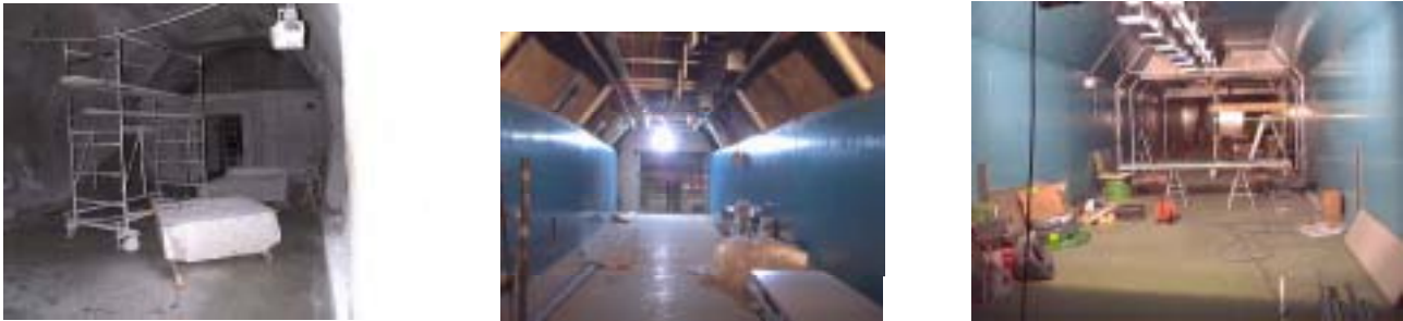
Fig 9-10-11 May 04, December 04 and May 05 pictures of BAM site work in progress.
