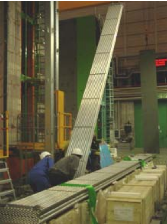
Installing one HPT module
