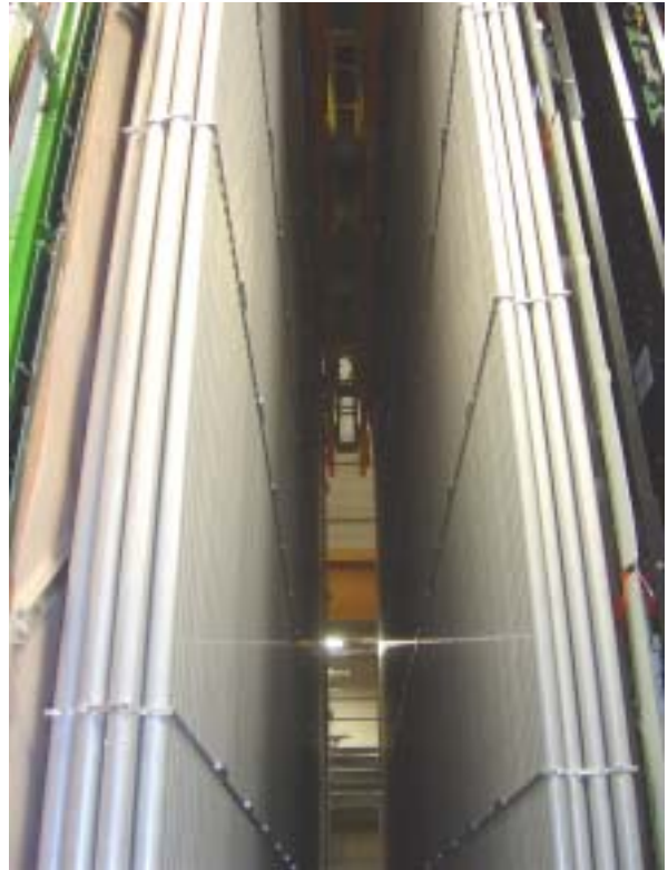
HPT planes 1 and 2 installed
