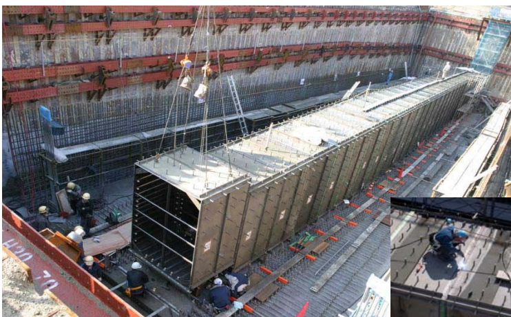
Figure 2.18: The 50 meter iron tunnel
