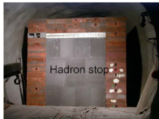
Hadron stop installed
