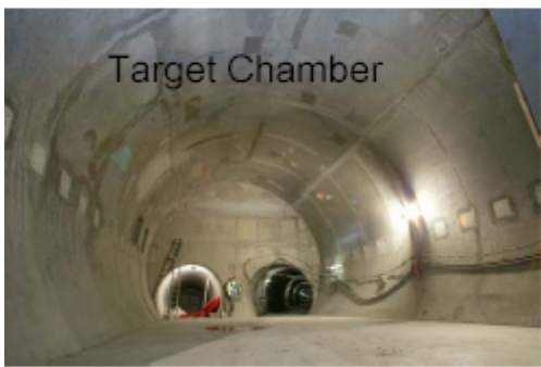
Civil engineering completed
