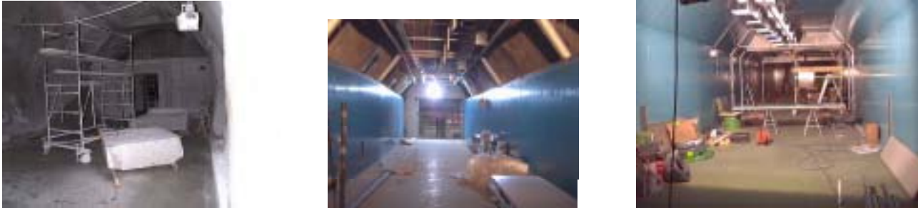
Fig 9-10-11 May 04, December 04 and May 05 pictures of BAM site work in progress.
