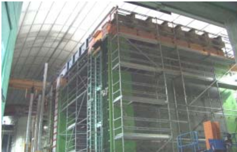
Fig.1: The OPERA magnets and support structures in May 2005. The support for the back arch is visible in the lower right corner.
